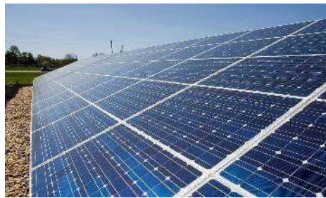
Figure 2 – Typical Photovoltaic Array
